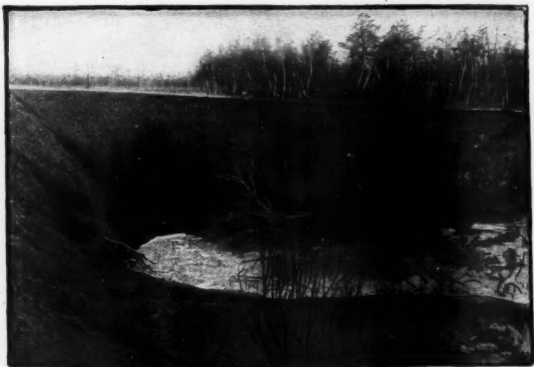
"THREE HUNDRED FEET BELOW THE FIRE HAD EATEN OUT THE PILLARS OF THE MINE, AND A CAVE-IN FOLLOWED."
